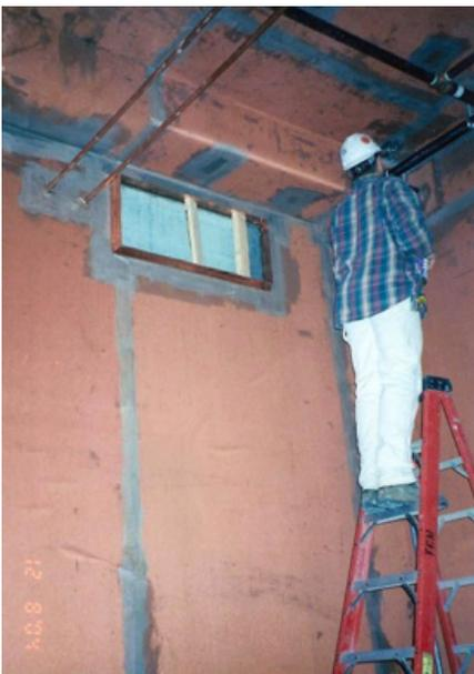
Typical interface required for door or window installation (wiring is temporary)
