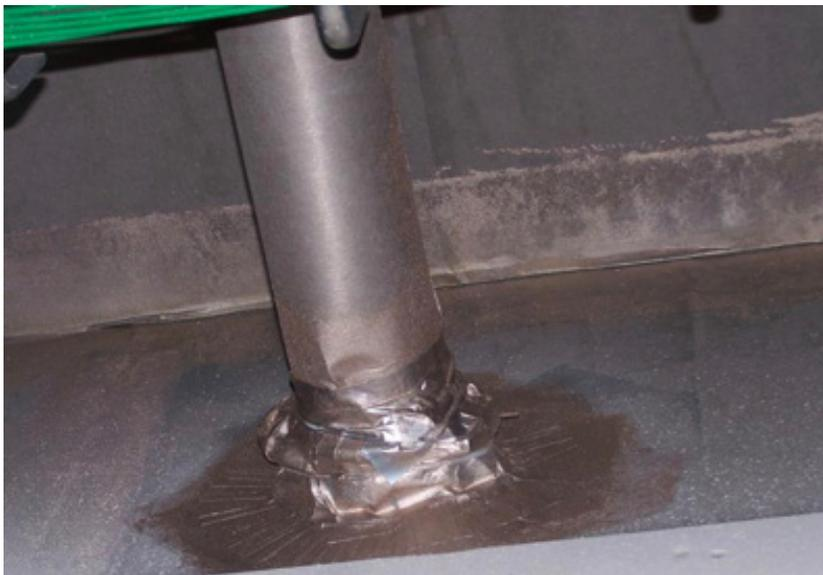
Floor covering with method of shielding a PVC drain pipe
