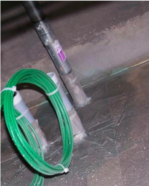
**Non-conductive pipe waveguides for fiber optic cable, with a copper pipe penetration.**
