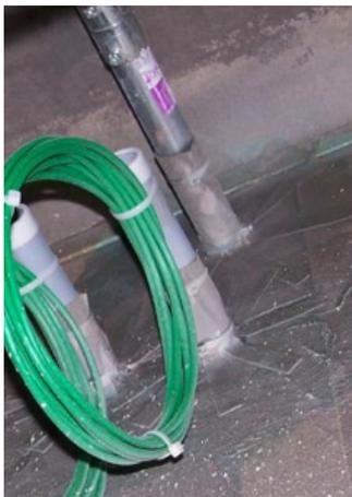
**Non-conductive pipe waveguides for fiber optic cable, with a copper pipe penetration**
