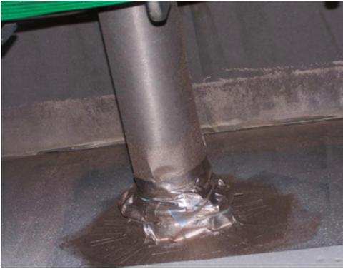
**Floor covering with method of shielding a PVC drain pipe**
