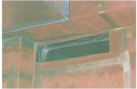
**Cut out prepared for mounting HVAC honeycomb filter**
